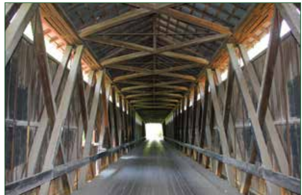
Interior view of the Dick Huffman Covered Bridge, a Howe timber truss originally constructed in 1880, located in Putnam County, Indiana.
