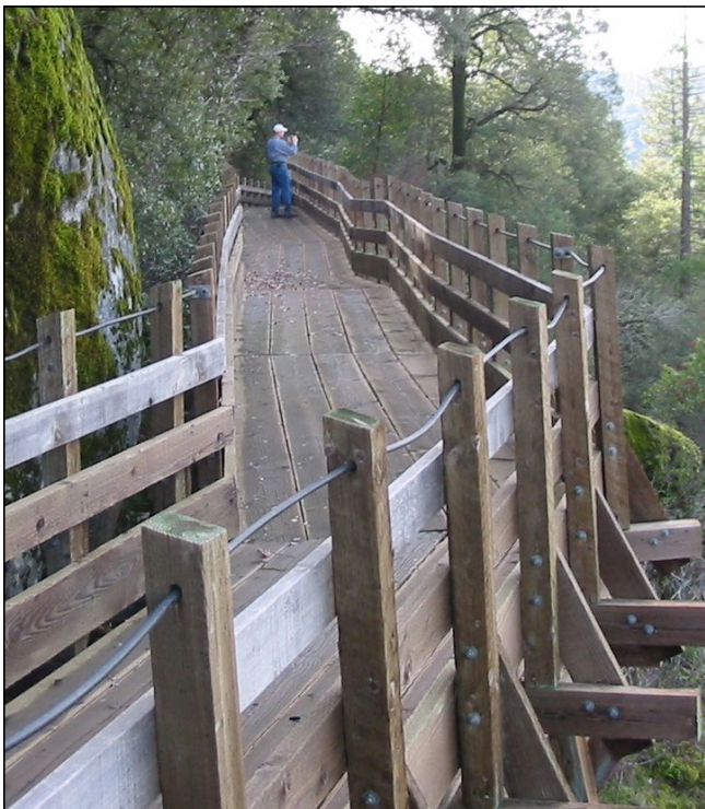
Figure 1. Treated lumber is often used where it is critical that the wood contain enough preservative to prevent damage from decay and insects.
