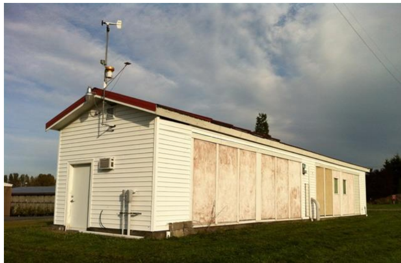
Figure 2. NET facility viewed from the southwest
