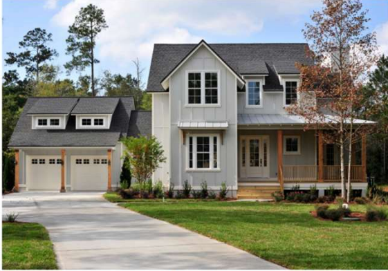
Owner/builder Scott Murray's desire for a home with height and curb appeal led to his decision to build a raised wood floor system that is "characteristic of the historic architecture that I like."
