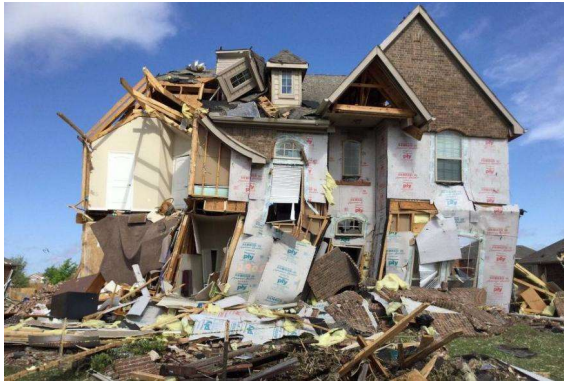
Poor load path
